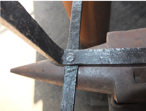
Fig. 21. A new rivet joining the frame.
