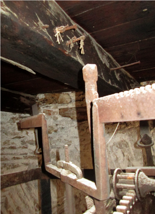
Fig. 28. In this photograph, taken before the refurbishment of the Ivron clock, the two nails used to suspend the foliot, which Riley had observed in the 1880s, are still in place.
